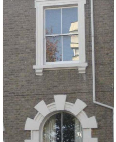
Traditional windows in The Waldrons Conservation Area. Above left: timber-framed with leaded detailing. Above right: timber sash with lugged architrave moulding sits above an arched window opening with mouldings including a keystone and stucco voussoirs.
