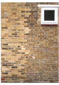
Photograph illustrating a poor matching of bricks for an extension with that of an existing building
