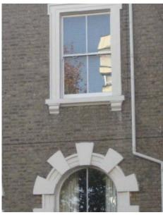
Traditional windows in The Waldrons Conservation Area. Above left: timber-framed with leaded detailing. Above right: timber sash with lugged architrave moulding sits above an arched window opening with mouldings including a keystone and stucco voussoirs.
