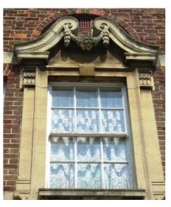
Decorative stone window surround of a timber sliding sash window in the Church Street Conservation Area. Stonework includes an architrave, pilasters and a voluted broken pediment linked by a swag.
